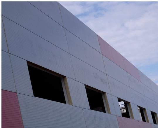
*Protection film was only stripped off after significant on site ageing. Glue residues are difficult to remove from the coil-coated surface*
