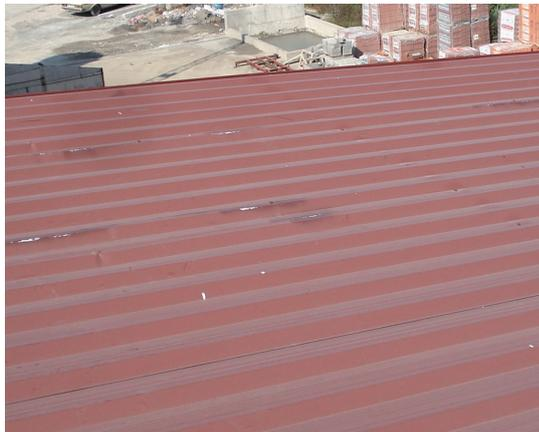
*Repainting is easy but some simple rules need to be followed. This is the aspect of a roof which has been poorly repainted*
