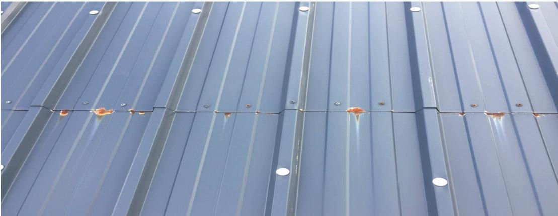
*Panels were unnecessarily cut on site and cut edges were not properly treated*
