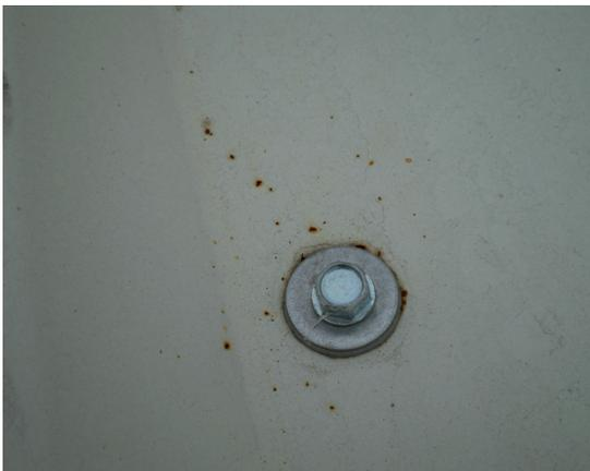
*Visible spot corrosion can happen when a coil-coated panel is drilled on-site if the metallic debris are not removed*
